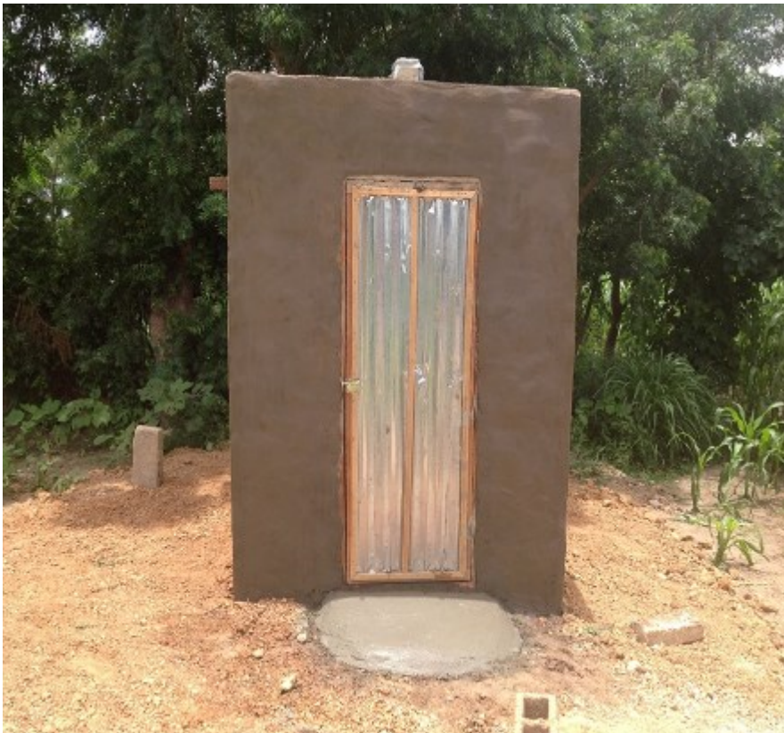
A single pit VIP latrine built for vulnerable people by masons during the training.
